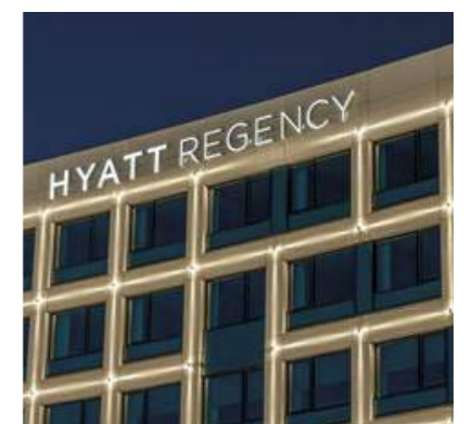
9 Custom fixtures are installed
